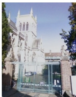
Forecourt Gate (with view of Chapel)
